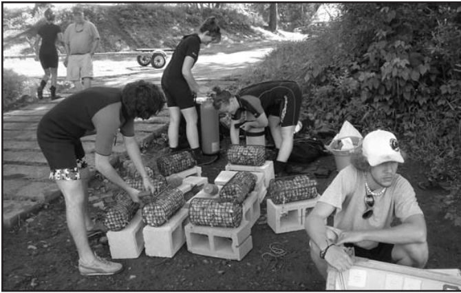
Interns preparing rock baskets for placement in the river.
