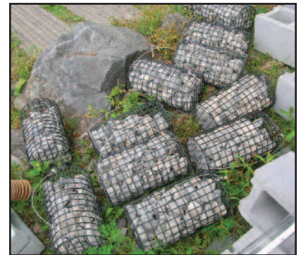
Rock baskets on bank of Susquehanna ready for submersion
