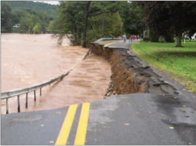
Section of Wallis Run Road collapsed in Lycoming County
