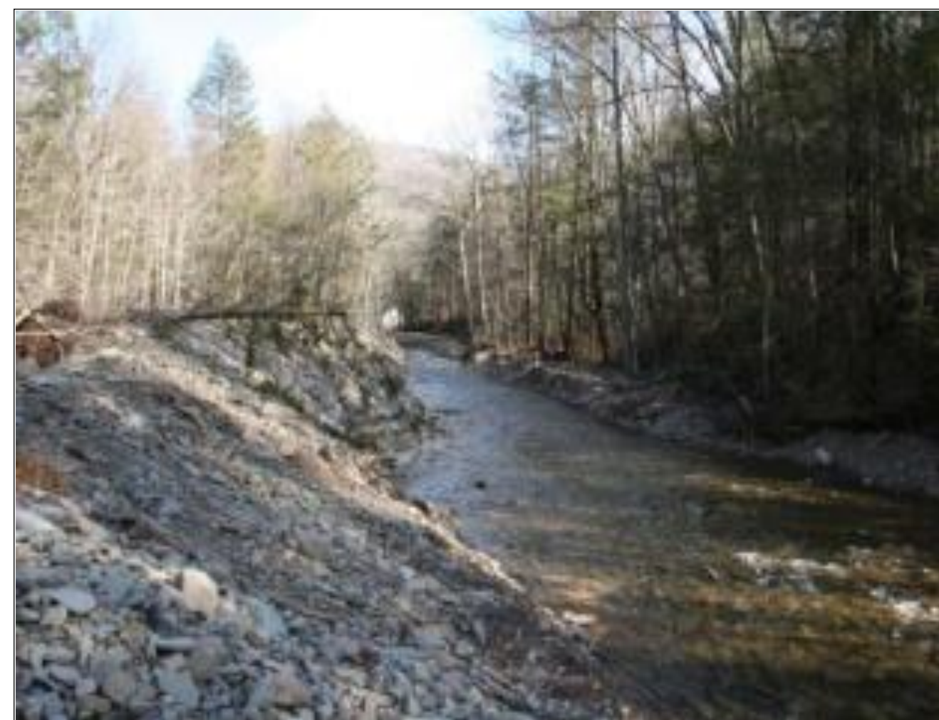
Figure 1. Cleaned site at Fishing Creek.
