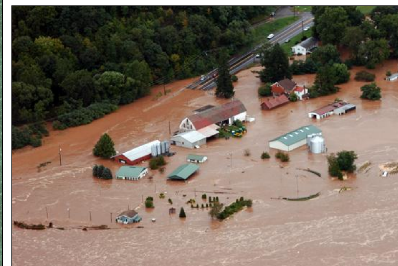
Figure 5. Overhead view of flooding near the mouth of Loyalsock Creek. The normal creek bed is over 500m away from the green barns off to the bottom right. (Photo: Williamsport Sun Gazette)
