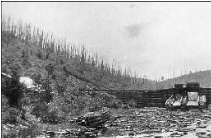
Splash Dam on Six Mile Run
